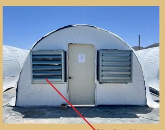
Exhaust fans push hot air out of the greenhouse to assist in cooling the space, as well as adding humidity. Light traps on the fans keep light from entering the house when blackout tarps are tricking the plants into producing flowers.
